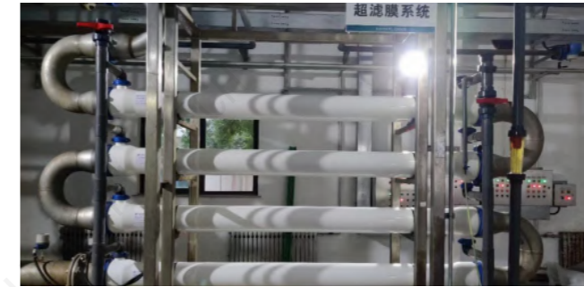
A Landfill Leachate Project in Weihai
