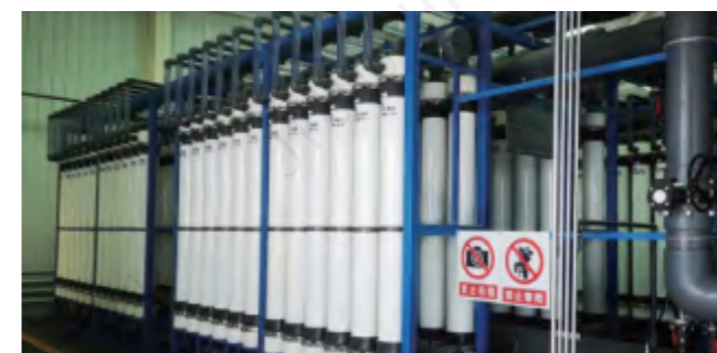
Lithium Extraction Project from a Salt Lake in Qinghai
