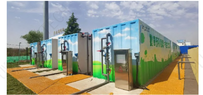
Lianyungang River Regulation Project
