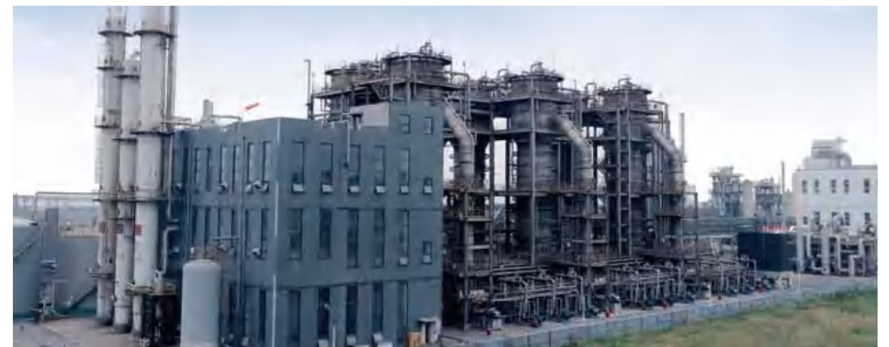
A ceramic membrane separation coupled fermentation process system for an annual production of 45000t/a fuel ethanol in a certain enterprise in Hebei Province.
